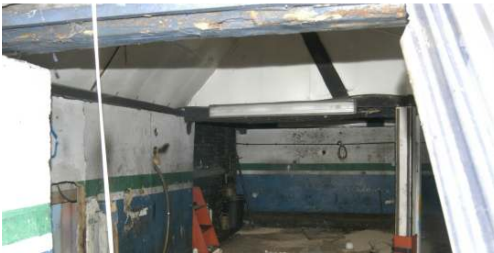
Figure 20: Central truss partially visible showing panelling either side of queen post
