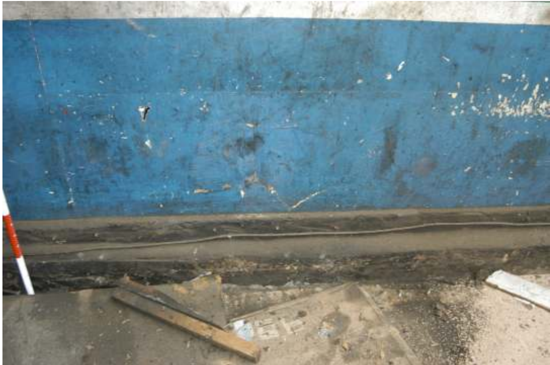
Figure 13: Timber sill beneath eastern wall
