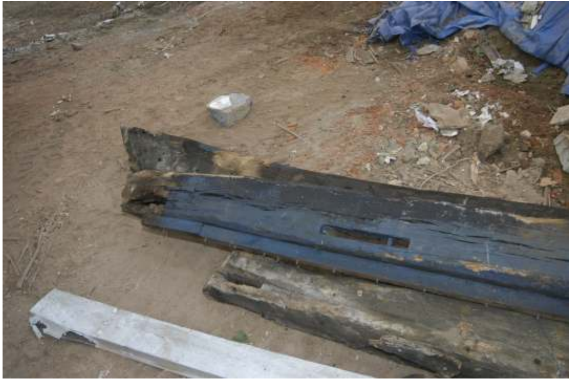
Figure 23: Terminal ends of long timbers following demolition
