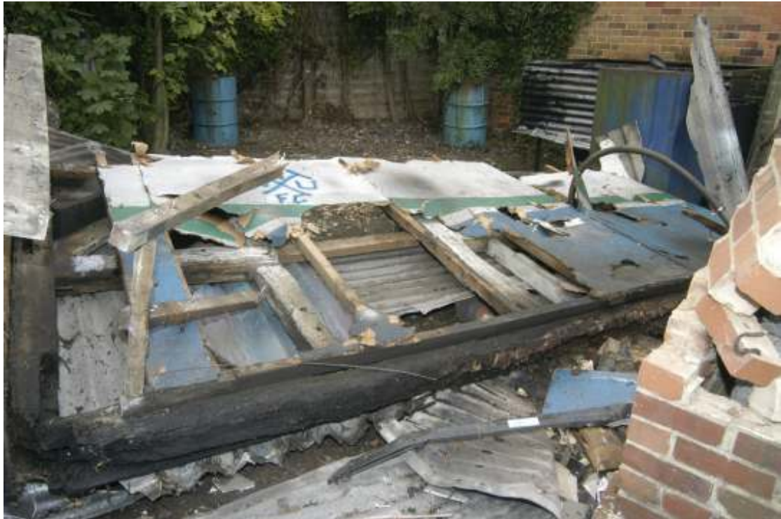
Figure 11: The north wall following demolition, part of the sill clearly visible
