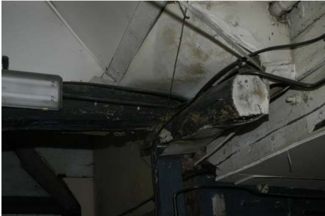
Figure 17: Wall plate truncated when new garage constructed
