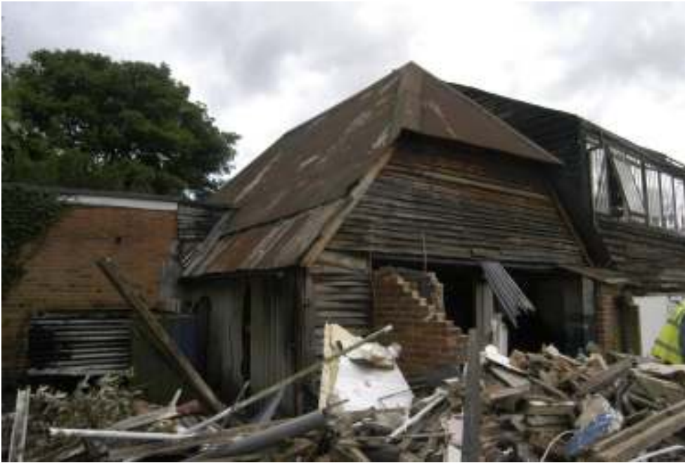
Figure 3: The barn prior to demolition, NW elevation
