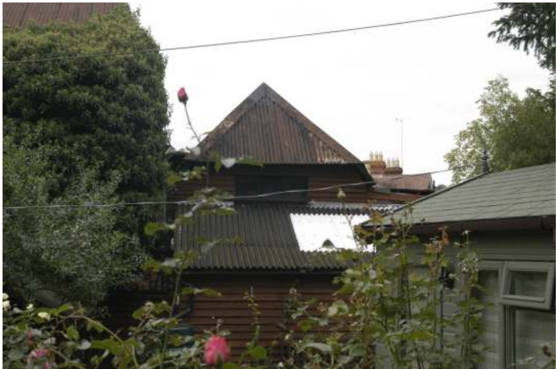
Figure 6: East elevation of barn
