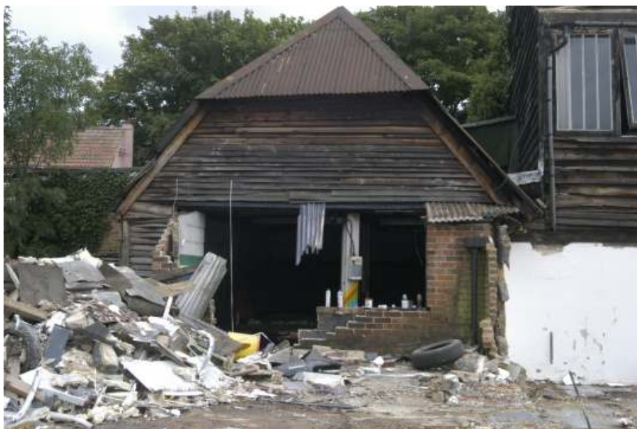
Figure 4: West elevation of barn
