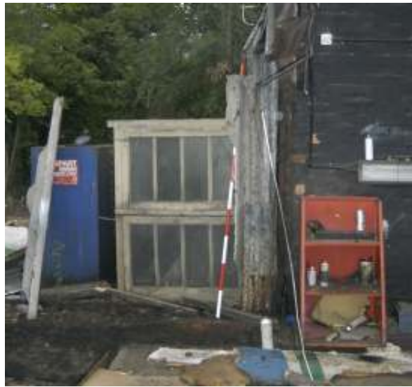
Figure 9: North wall following demolition
