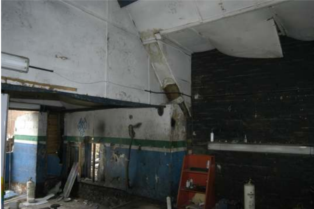
Figure 7: Interior, northern elevation
