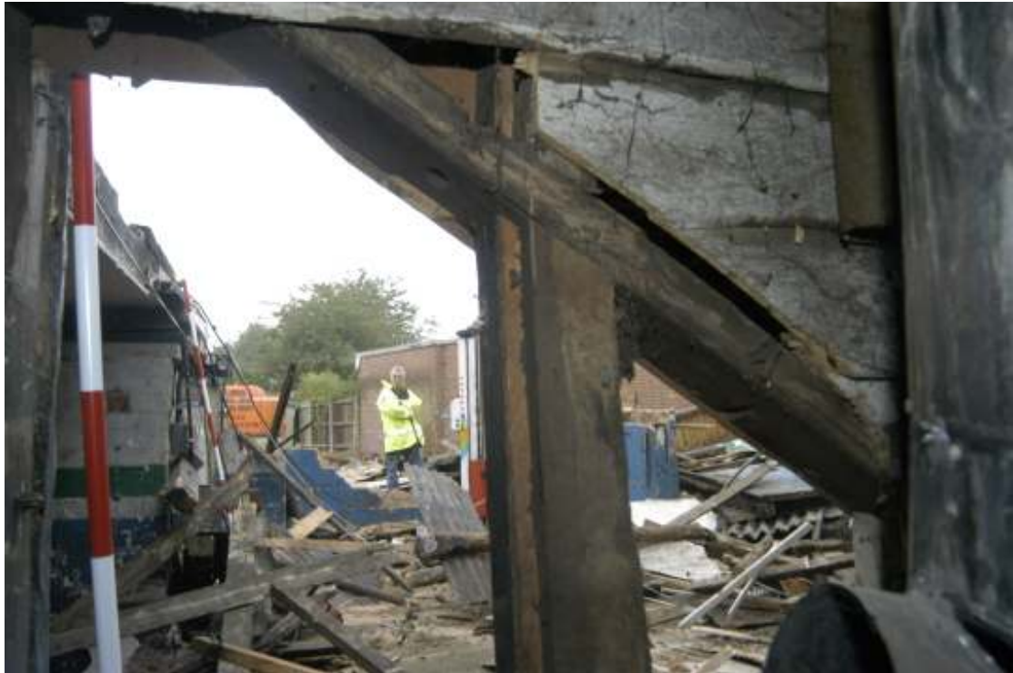
Figure 15: Cut-out in east wall showing timbers and possible original cladding
