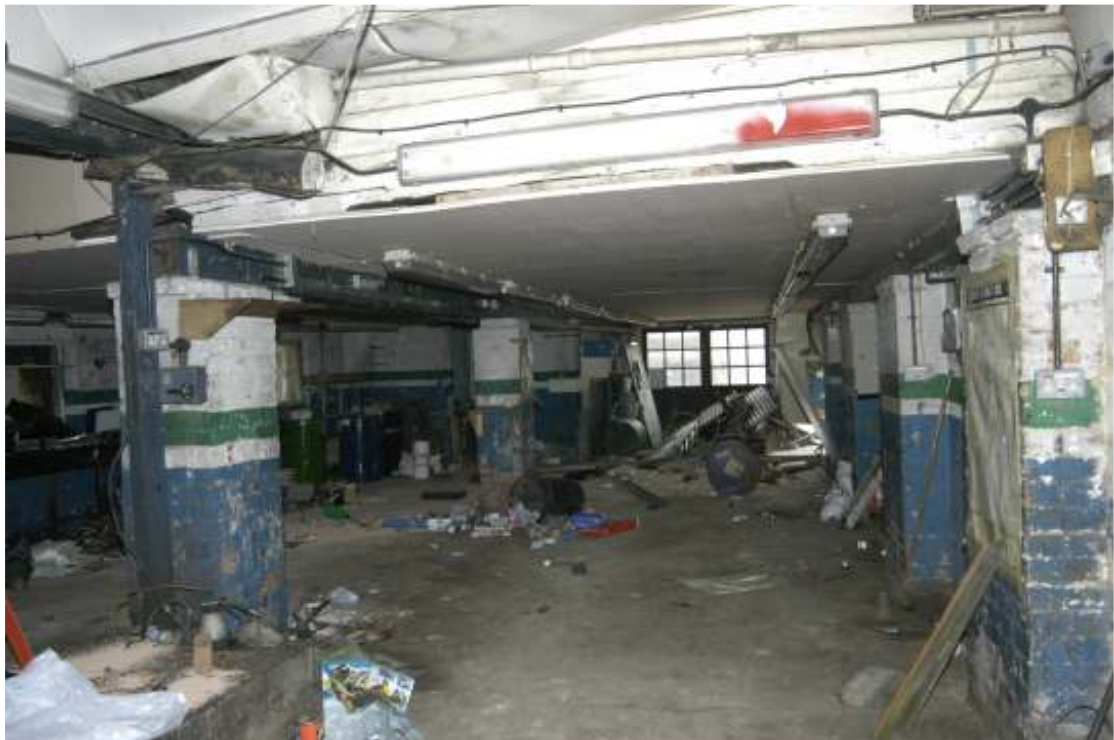
Figure 16: South of the barn, the main workshop
