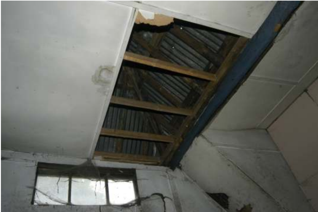
Figure 21: Roof panelling removed showing original timbers above
