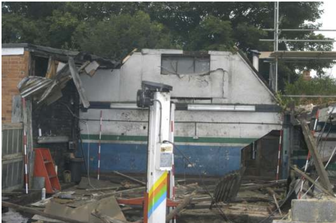
Figure 12: The eastern wall of the barn
