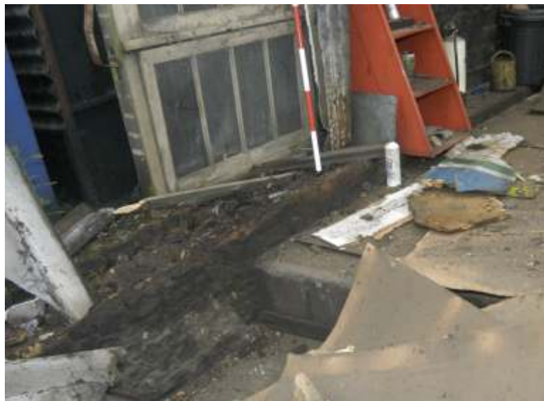
Figure 10: Timber sill beneath the north wall
