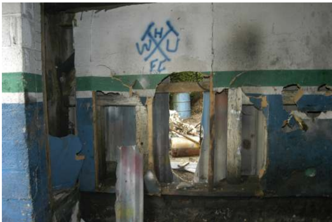
Figure 8: North wall detail, showing original timbers
