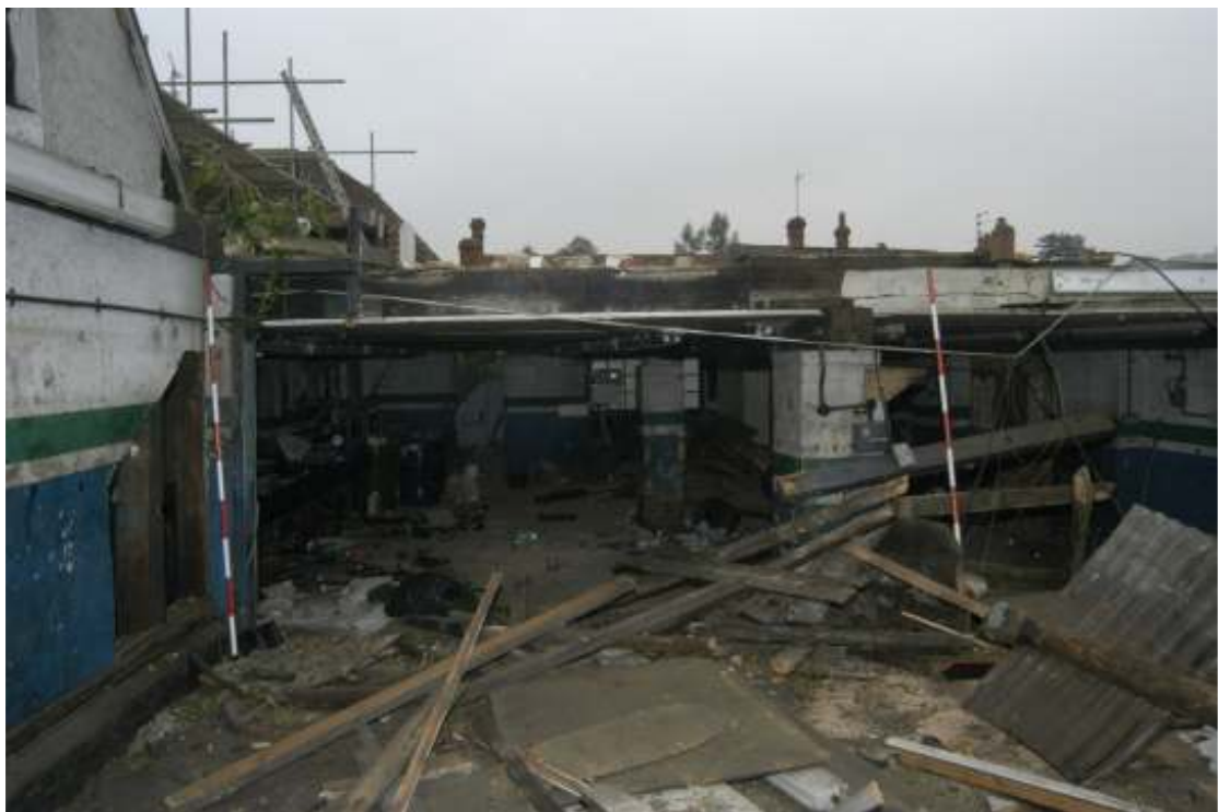
Figure 18: South elevation following demolition of barn
