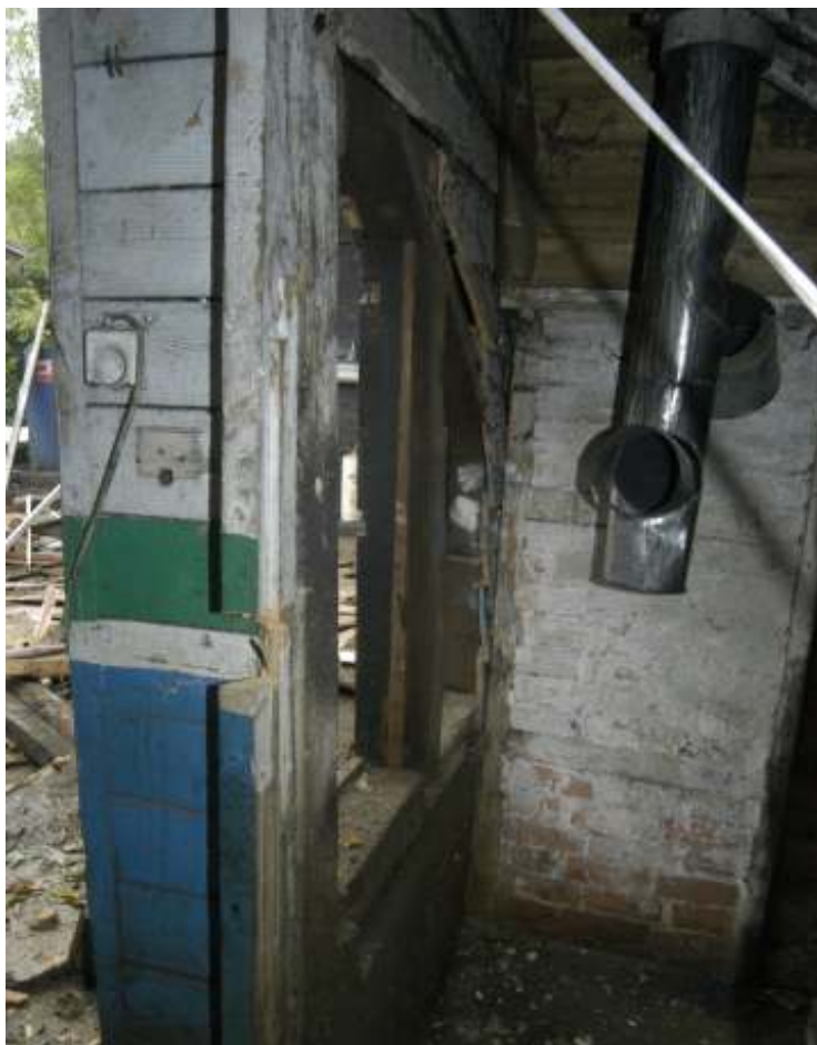
Left: Figure 14: Boiler recess, east wall
