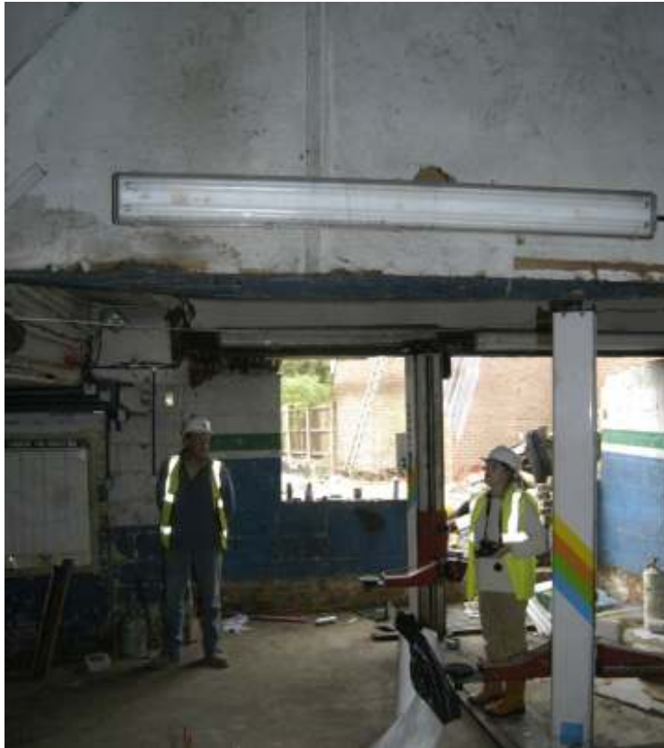
Figure 19: West elevation of barn
