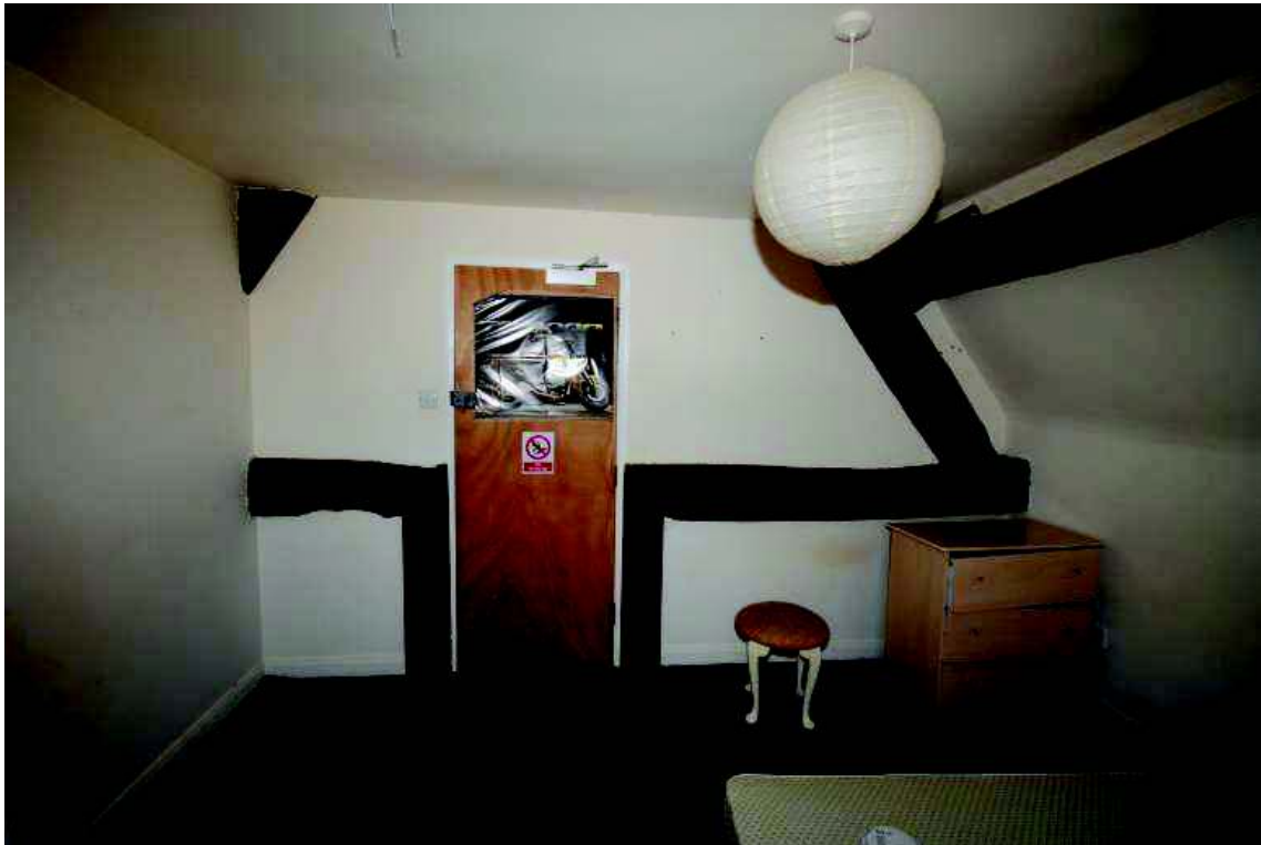
Plate 35: Roof truss, first floor north, 3A
