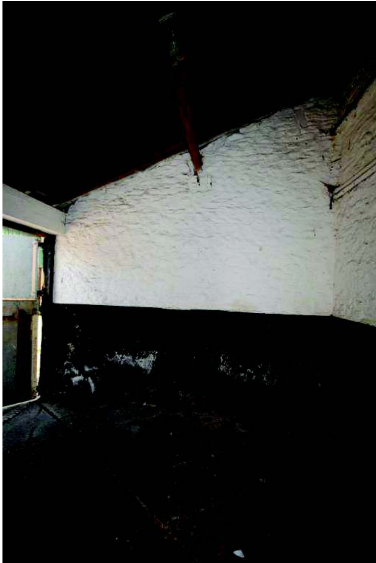
Plate 23: Southern wall and roof structure, 2B, viewed from north
