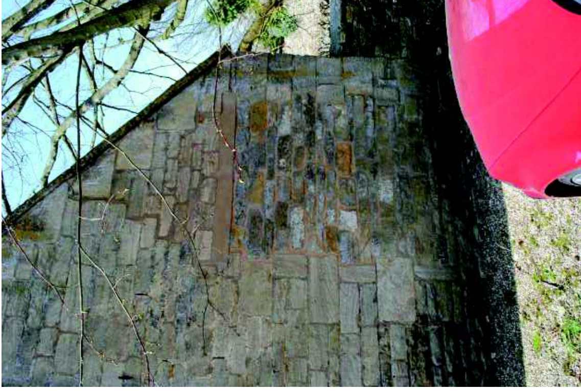
Plate 10: Detail of blocked doorway, eastern elevation, building 1
