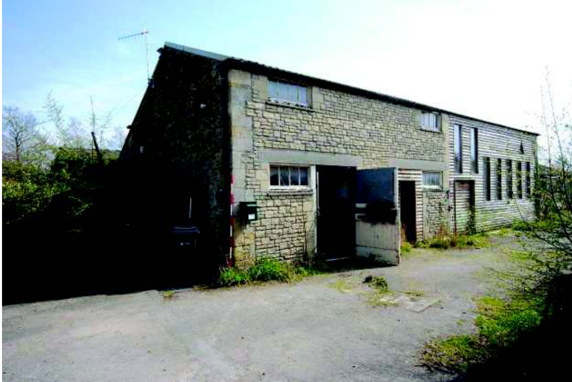
Plate 11: Northwest aspect, building 2A
