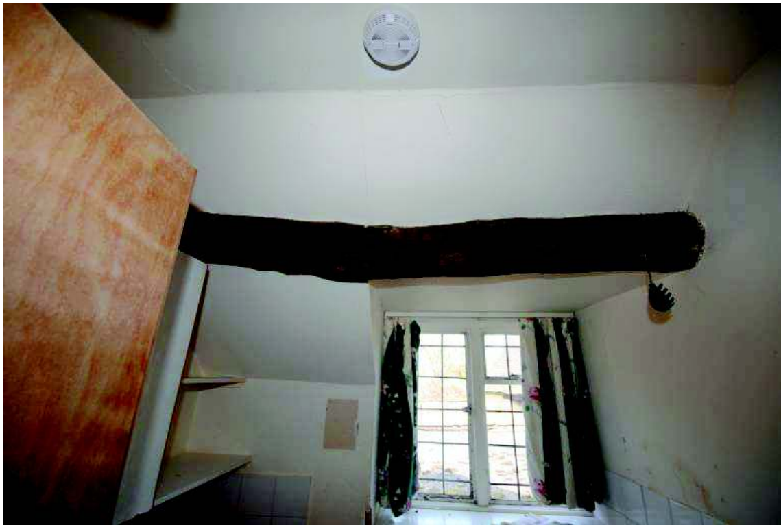
Plate 48: Detail of purlin, first floor kitchen, 4A
