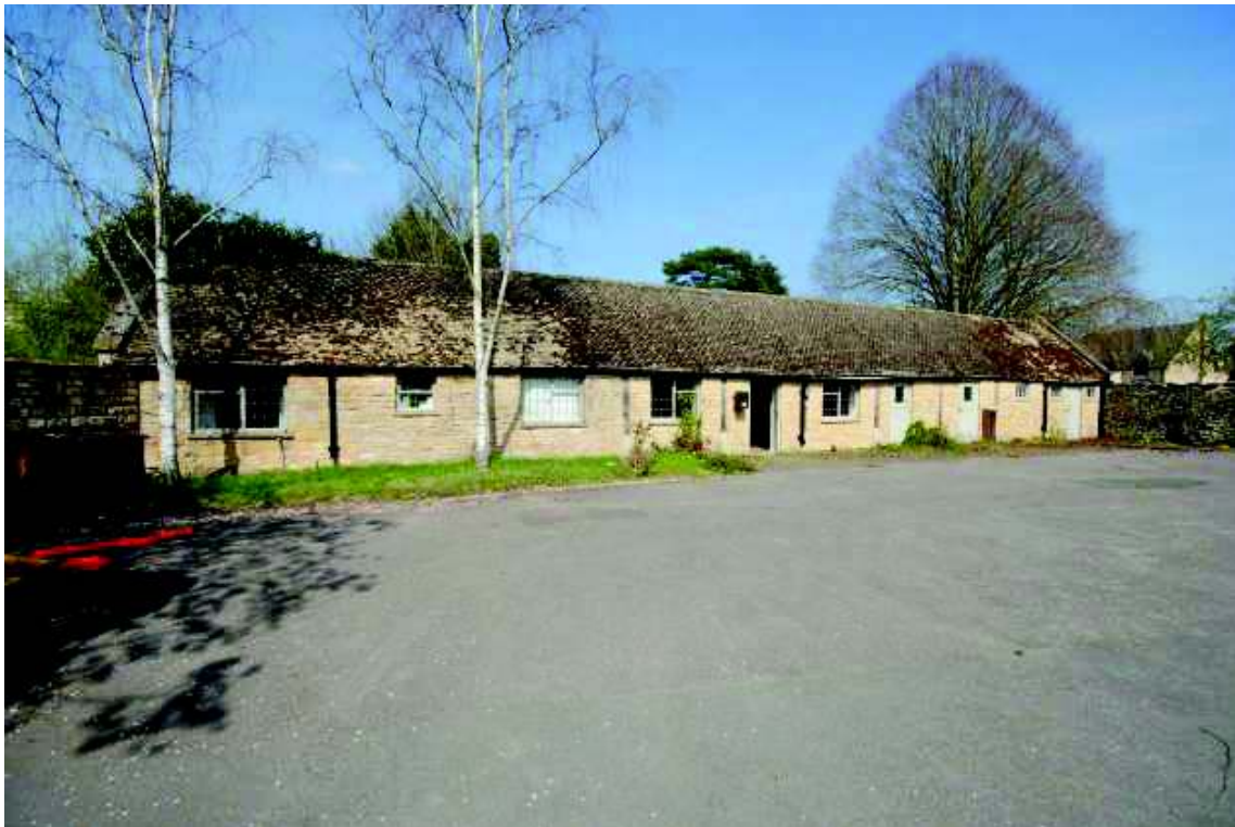
Plate 1: Southern elevation, building 1
