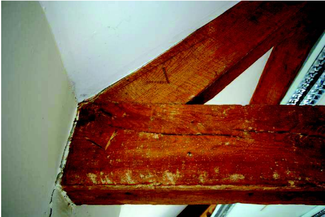
Plate 6: Internal carpenters' marks, building 1 (manipulated image)
