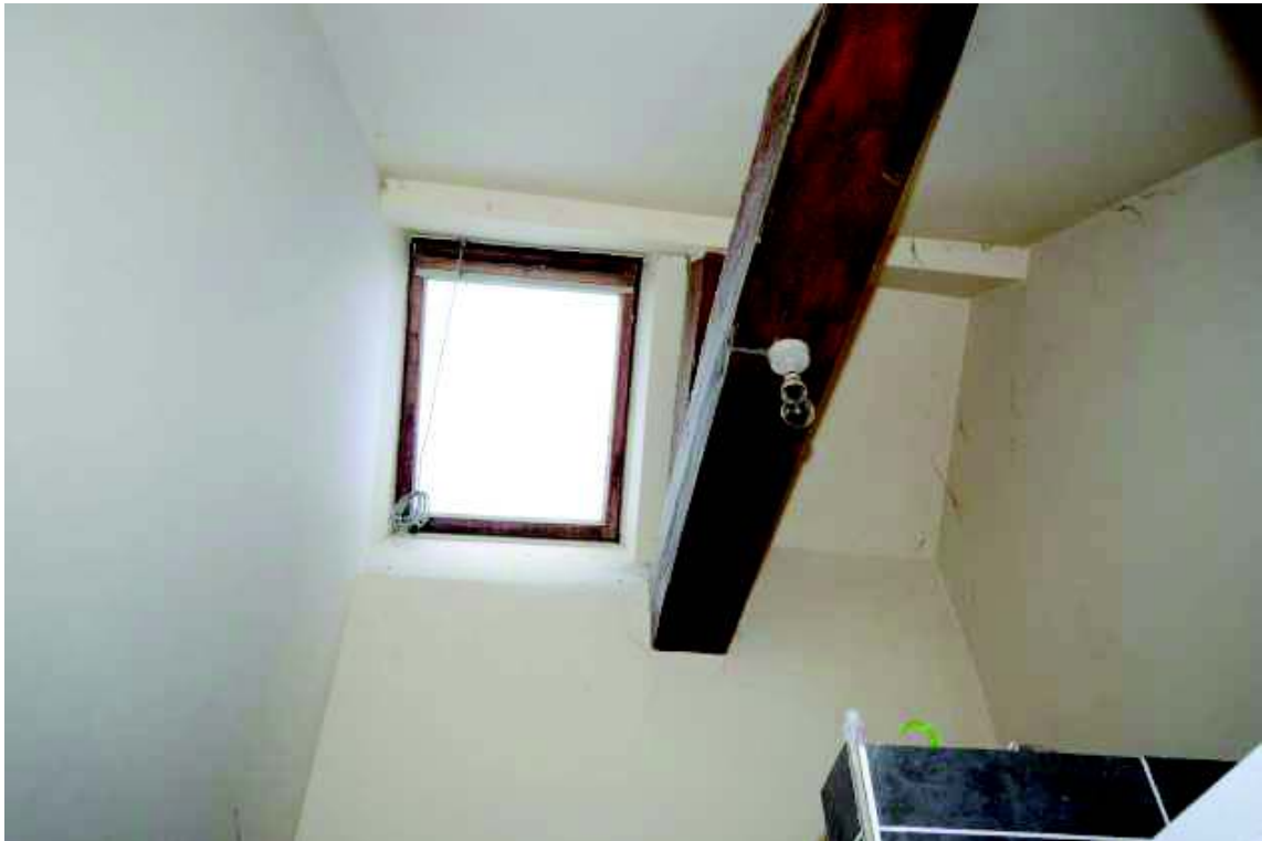
Plate 47: Timbers, ground floor bathroom, 4A
