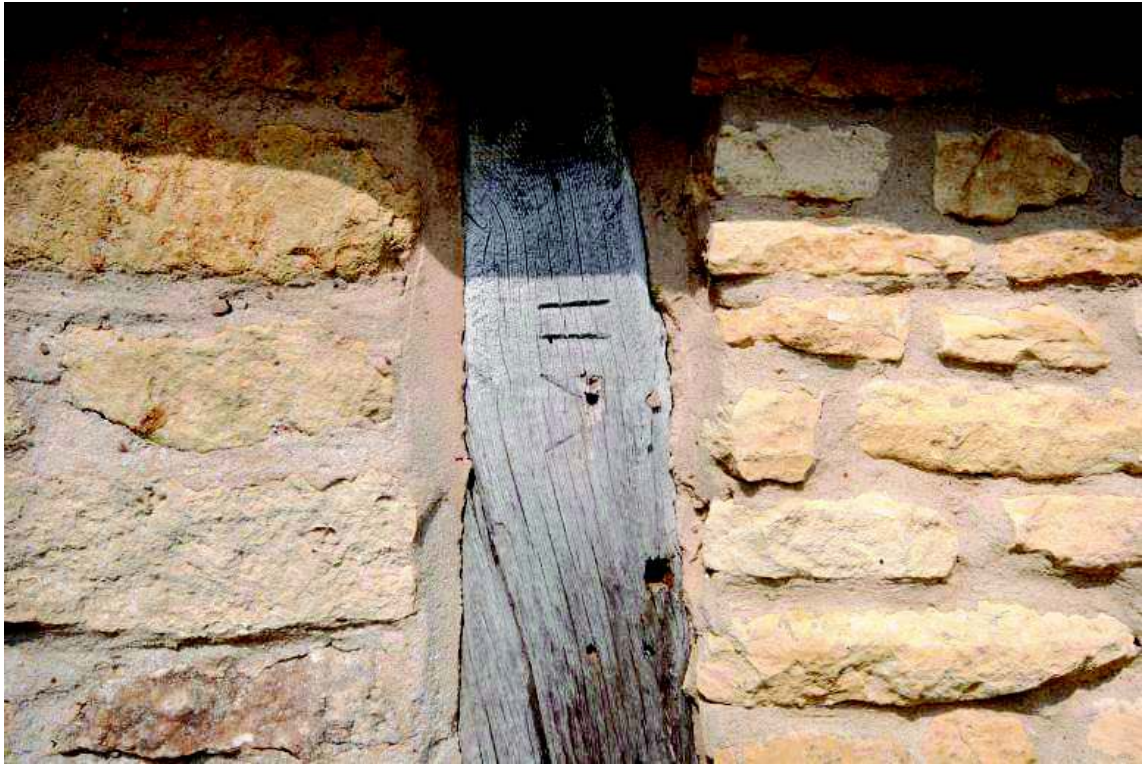
Plate 8: External carpenters' marks, building 1
