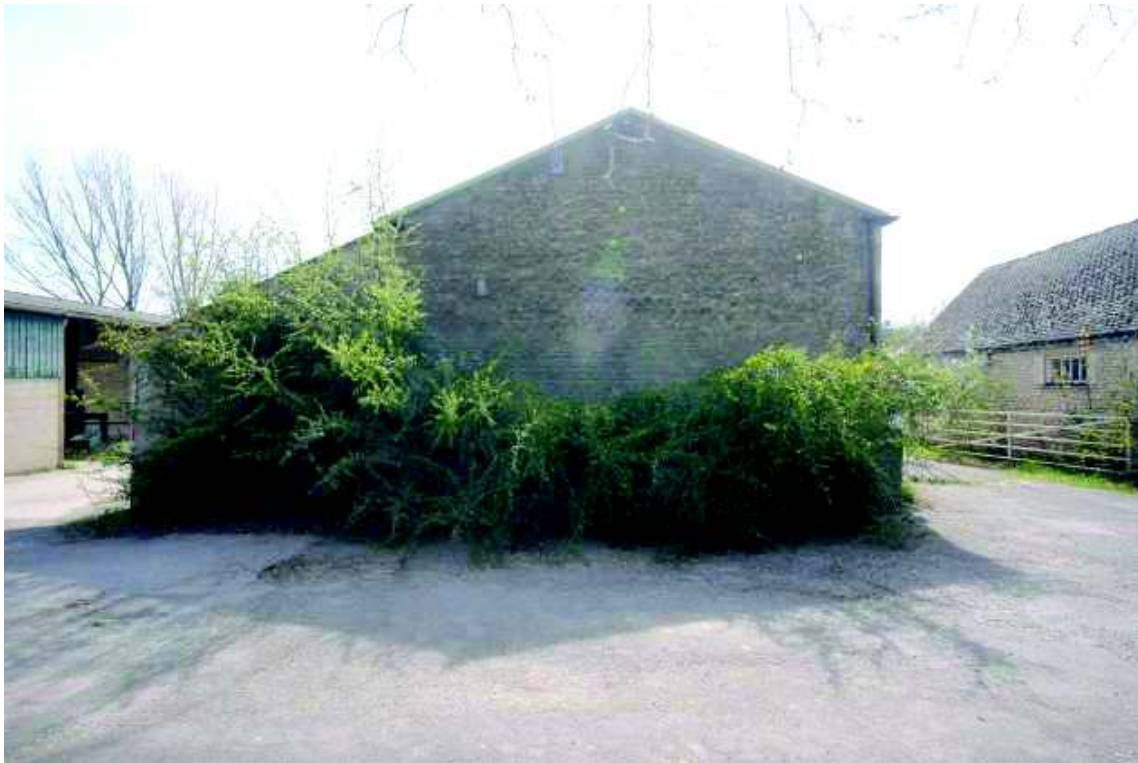
Plate 12: Northern elevation, building 2A
