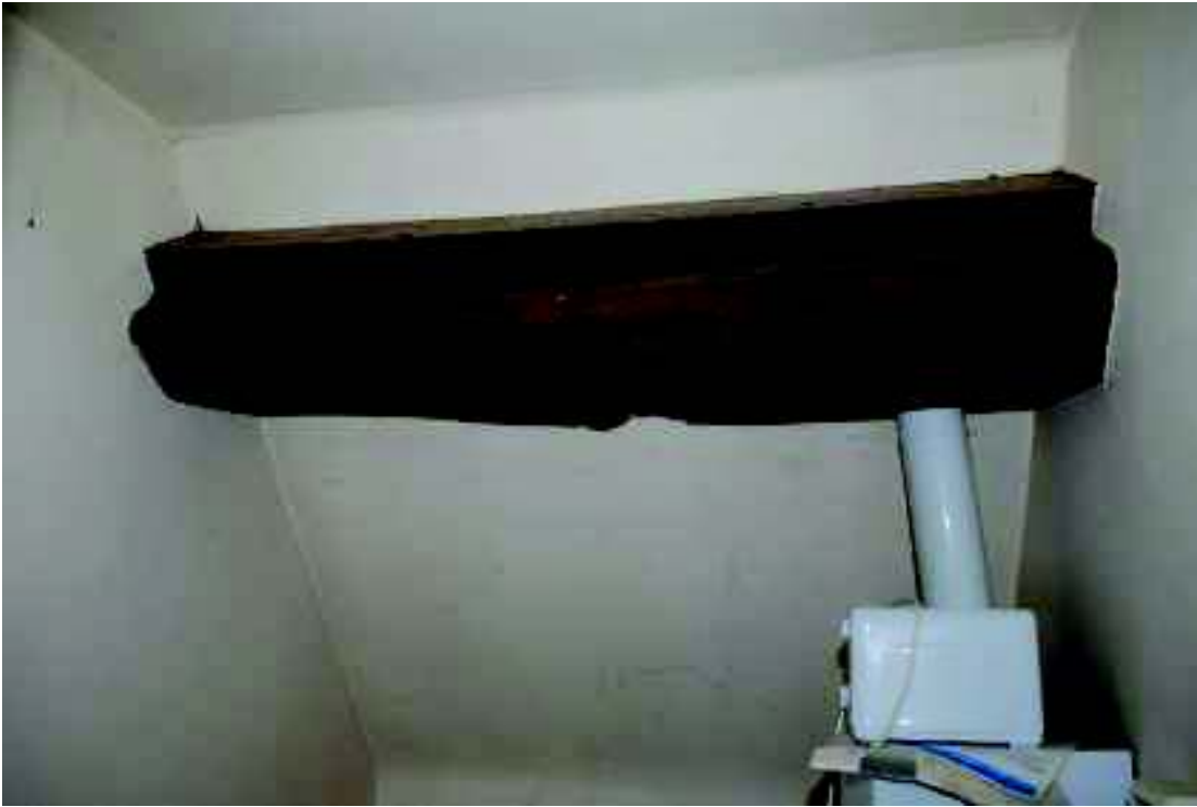
Plate 36: Lower purlin with modern timber above, cupboard, landing east, 3A
