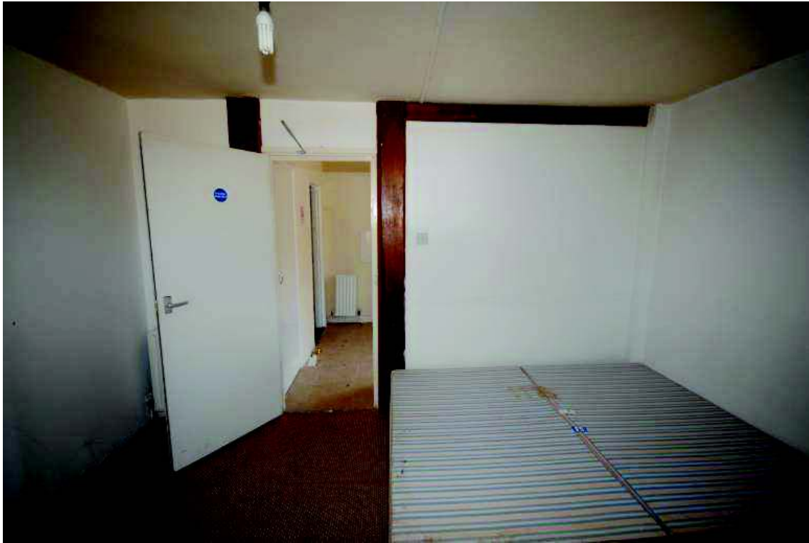
Plate 32: Modern timbers, ground floor, 3A
