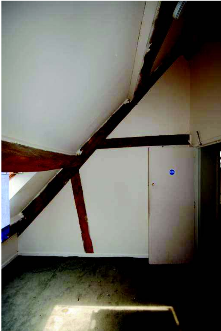
Plate 50: Detail of timbers, central bedroom, 4A
