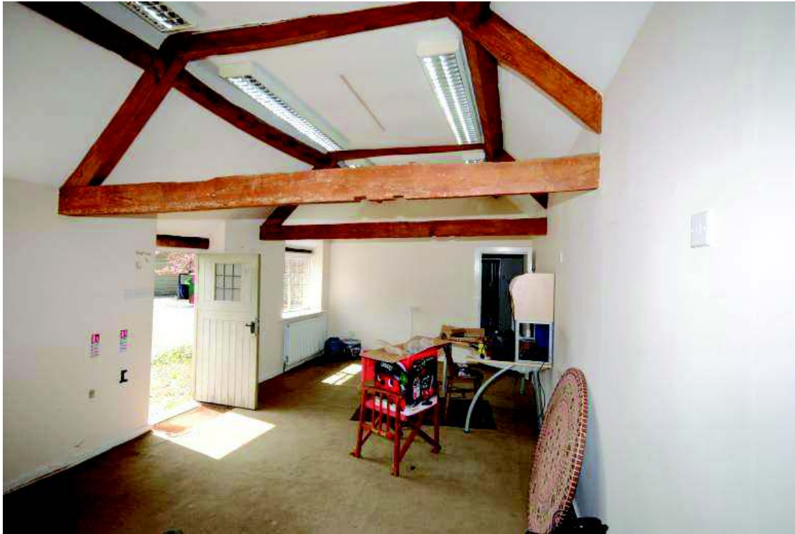
Plate 4: Detail of roof truss, central room, building 1
