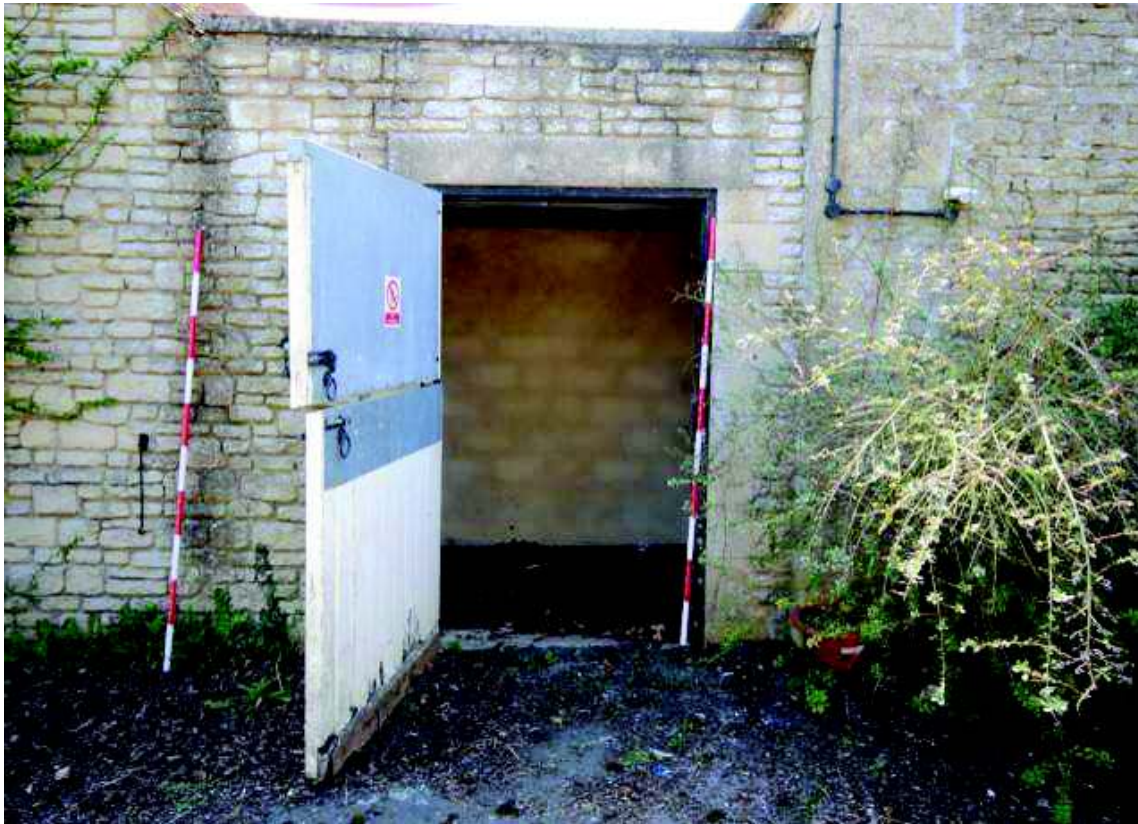
Plate 40: Northern door to 3E
