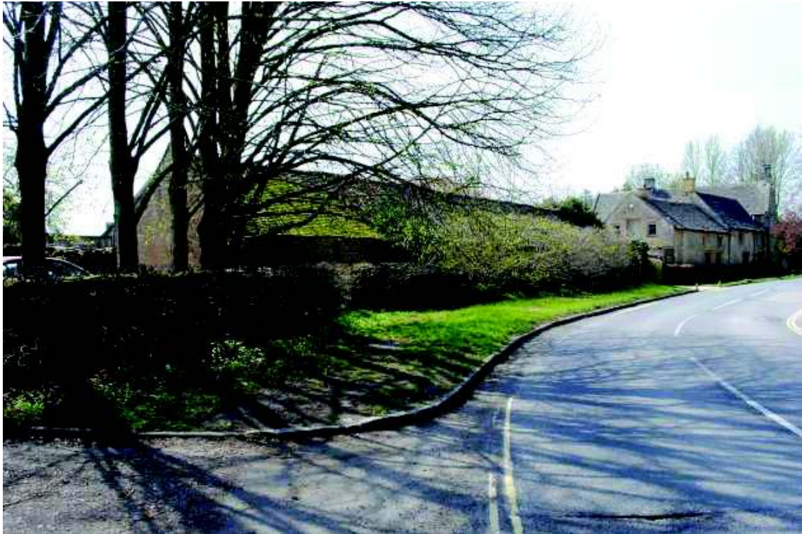
Plate 2: Rear (northern) aspect, building 1, viewed from road
