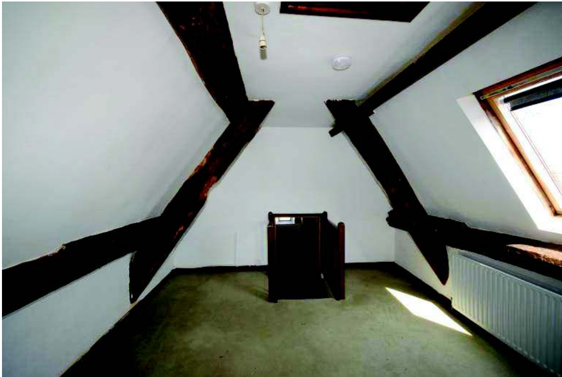
Plate 33: Northern aspect, first floor south, 3A
