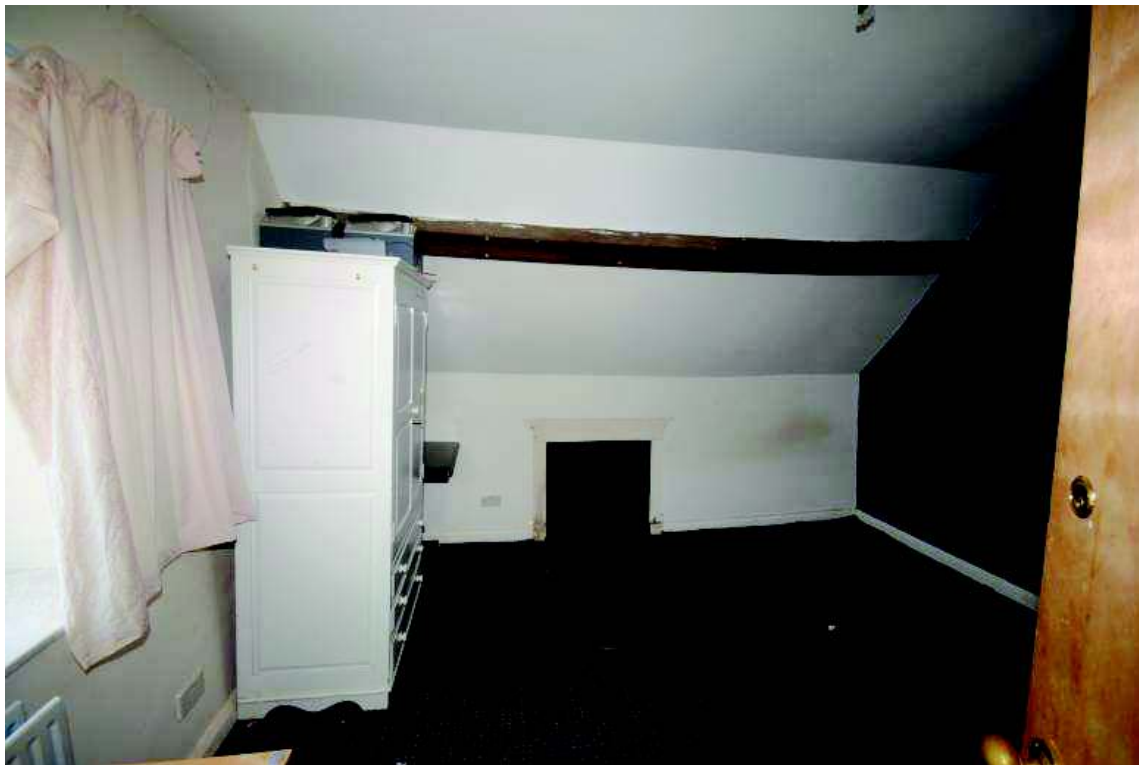
Plate 49: Detail of purlin, phase 1 bedroom, 4A
