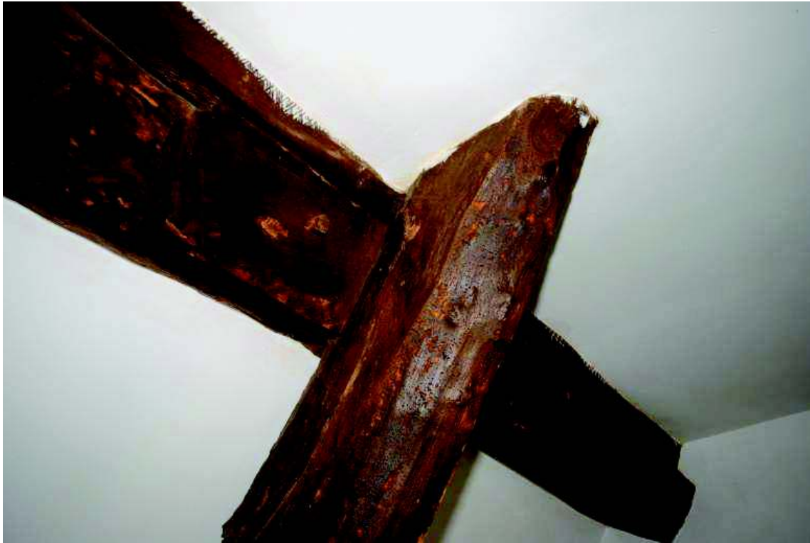
Plate 34: Detail of timbers, first floor south, 3A
