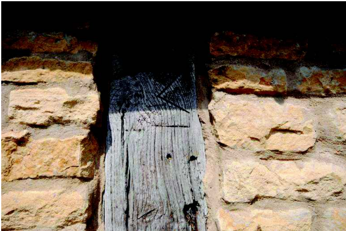
Plate 7: External carpenters' marks, building 1
