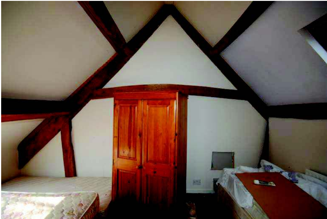
Plate 52: Detail of timbers, first floor west, 4A
