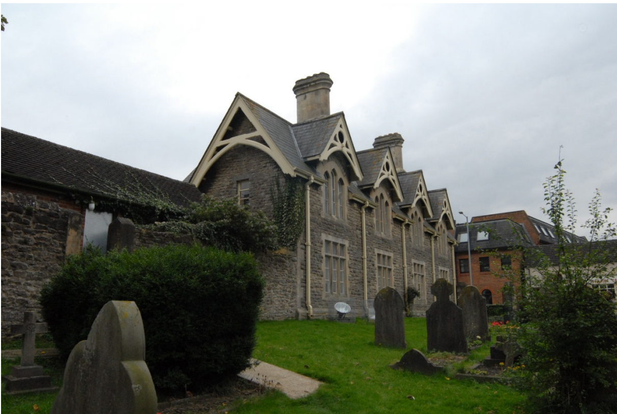
Plate 1: Almshouses, 27-30 Cricklade Street, Swindon
